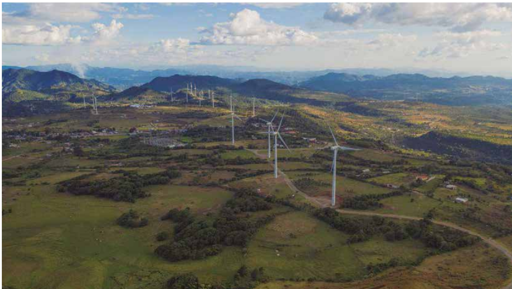
Wind Plant Cerro de Hula, Honduras
