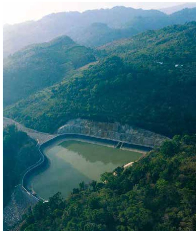
Hydroelectric Renace IV, Guatemala
